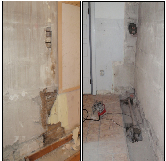
Sections of wall where plaster repairs were desperately needed (left); the hole left behind from steam pipe modifications (right).
