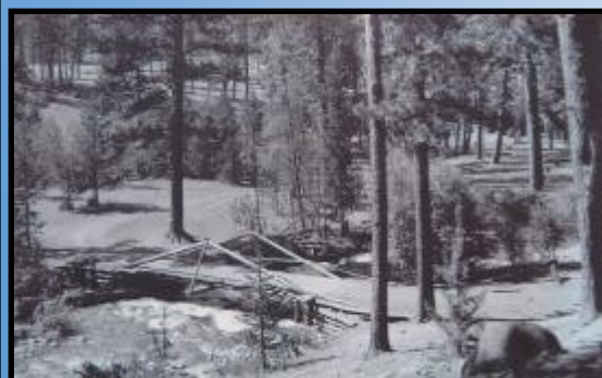
Tumalo Creek bridge at Shevlin Park, photo courtesy of the Bowman Museum
