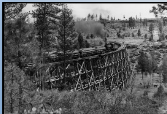
Railroad trestle over Shevlin Park
