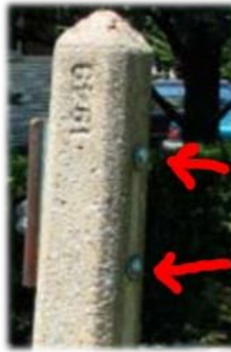
(L) Example of mounting bolt placement from the “Forgotten New York” website
