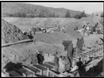
Camp Redmond enrollees pouring concrete walls along the main canal structure of the Deschutes Project. (National Archives and Records Administration)
