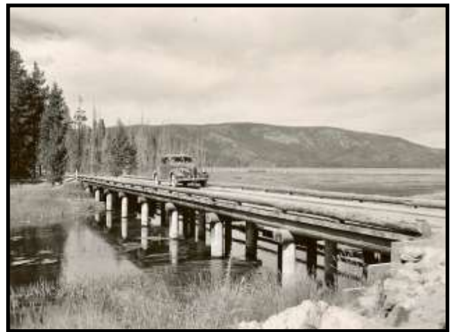
A CCC-built bridge crossing Paulina Creek with Paulina Lake in the background, 1935. (Forest Service)
