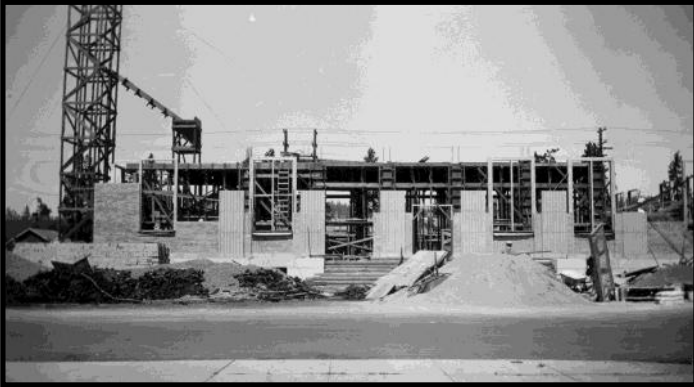
1932— US Federal Post Office Wall St entrance, first floor under construction.
